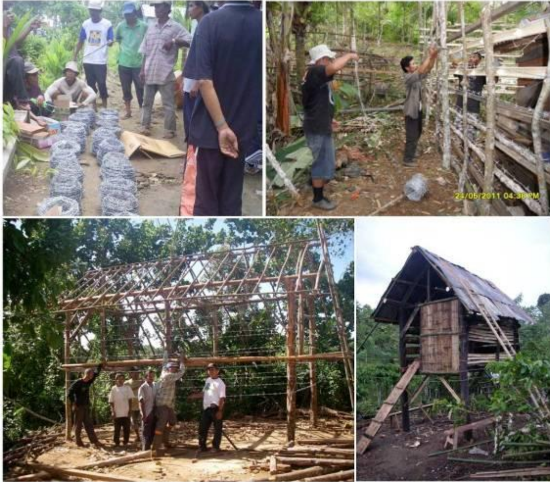
Figure 10: To reduce human-tiger conflict, WCS staff regularly work with villagers to construct tiger proof enclosures for domestic livestock. Such enclosures are deliberately inexpensive to construct and maintain and rely on simple, readily available materials such as barbed wire. Tiger proof enclosures range in size depending on local conditions. WCS has worked with local villages to construct hundreds of such tiger proof enclosures across the Leuser and BBS landscapes.
