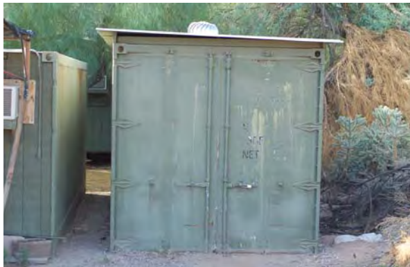
Figure 4. Original exterior doors before removal.
