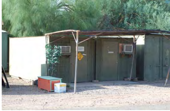
Figure 2. Wide view of MACC and its concrete pad stoop.
