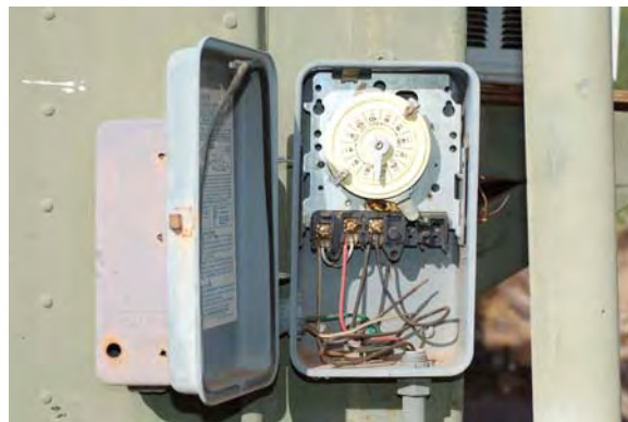
Figure 10. Pool timer used to program lights.
