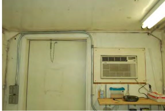
Figure 5. Inside view of front wall replacing swing doors
